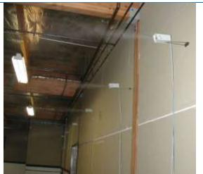
In this Application, Fog Nozzles are Placed about 8 feet or 2-1/2 Meters apart on one or more of the Warehouse Walls.
